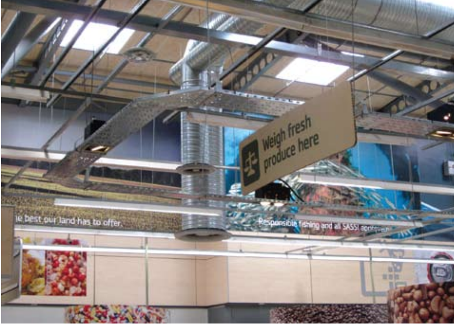
Pick n Pay on Nicol's use of natural lighting is energy efficient, as well as creates a relaxed and warm shopping environment for customers.
