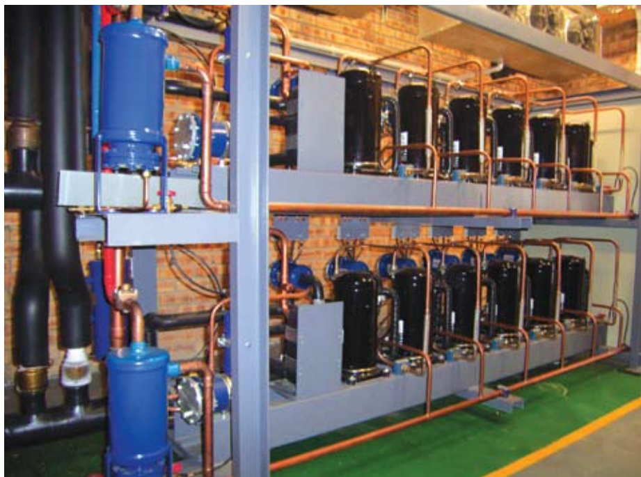
Scroll compressor rack with EVI. The heat exchanger for the rack is half the size of a compressor and is tucked away out of sight in this picture.
