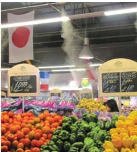
Timed overhead sprays keep the fresh produce cool, which helps the fruit and vegetables last longer.
