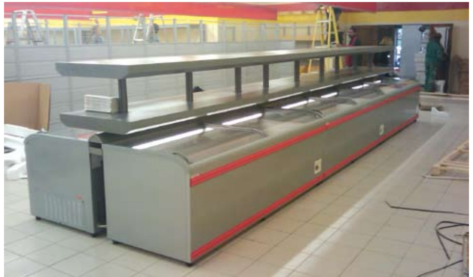
Removable glass lids keep the temperature constant and ensure that the product quality is consistent because of minimal temperature changes.
