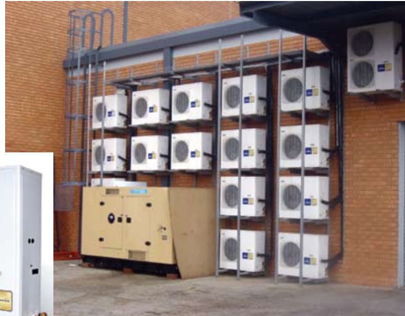
Refrigeration plant room on a wall! ZX units save valuable space. Here they are seen clustered neatly together.
