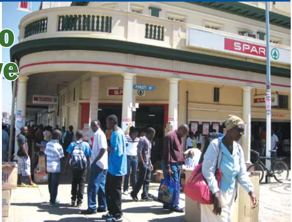
Permission had to be granted by the National Museums and Monuments of Zimbabwe so roll shutters could be added to the façade of the building in First Street Spar's expansion.
