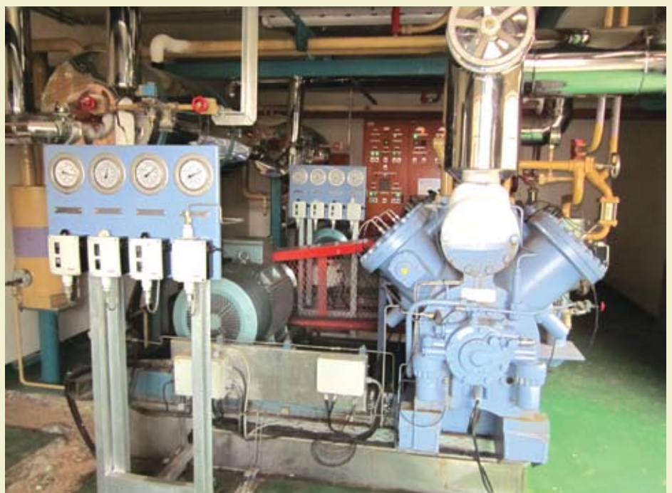
For MD of F. Dawood, Iqbal Faki, an efficient refrigeration system is crucial for the bottom line. This has been achieved by introducing mobile racking to their cold rooms; reducing energy waste with limited door entry and a strong management system.
