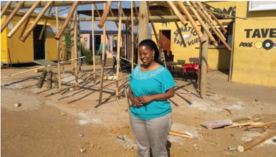
Lebo outside her Food Zone premises, shows the expansion with the construction of a new thatch boma. She uses empty food warmers on the outside tables to attract attention to her take-away offering to passers-by.
