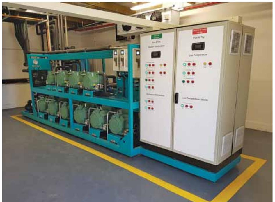
The CO<sub>2</sub> transcritical refrigeration pack was built by Sphere.
