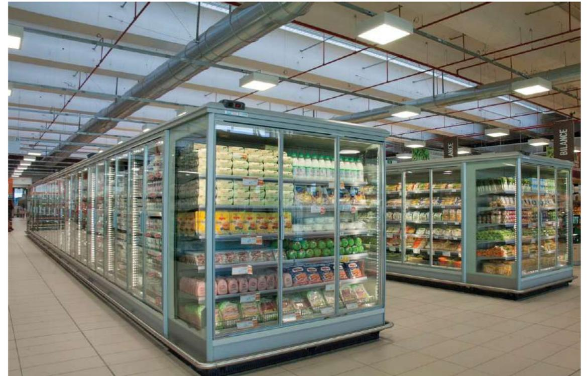
store. This is claimed the most power efficient refrigeration system. There are a number of other associated benefits. It offers the most stable cabinet temperatures with users claiming up to four days more shelf life in fresh meat as a result. With less than 1.8m of copper tubing and 3 kg of gas per cabinet there is little chance of a gas leak and little gas to lose if there is one .
