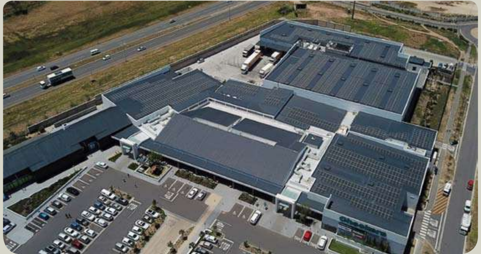
Checkers Sitari (Somerset West, Western Cape), one of the many stores that harness the power of the sun for their operations.
