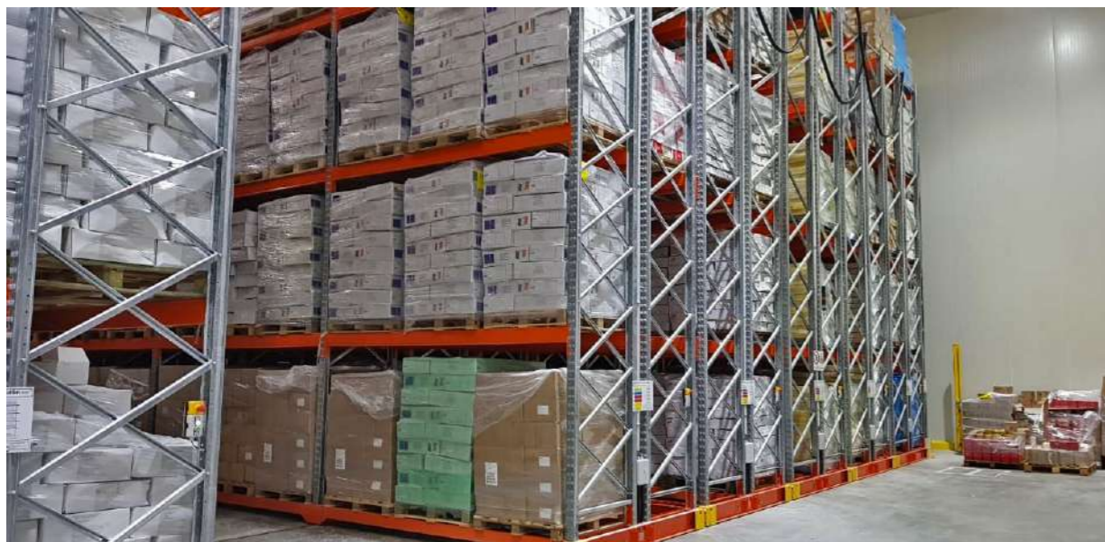
The freezer rooms are equipped with motorised racks that stack up to create more space.
