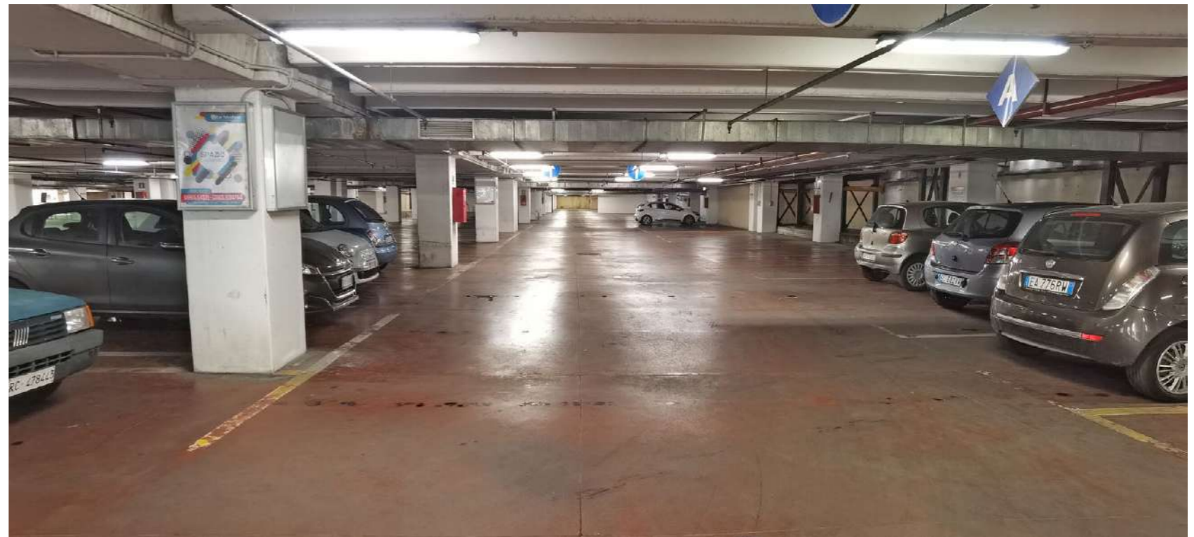
View of the large underground car park
